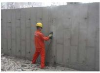
**Grinding**Suitable for creating a CSP-1 to CSP-3.
