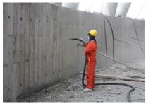
**Sandblasting** or **shotblasting** Suitable for creating a CSP-2 to CSP-8.
