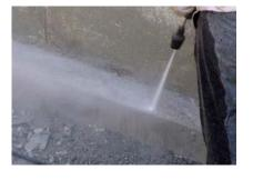
High-pressure water blasting (at least 350 bar) Suitable for creating a CSP-3 to CSP-10. In case there is formwork release oil on the surface, apply a suited detergent to the surface before cleaning with the water jet.
